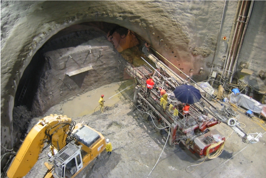
Special tunnel drill rig RODIO SR 510 inside the start shaft
